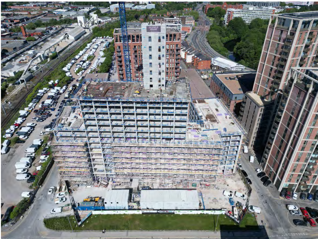
^ Oldfield Wharf signage in place
